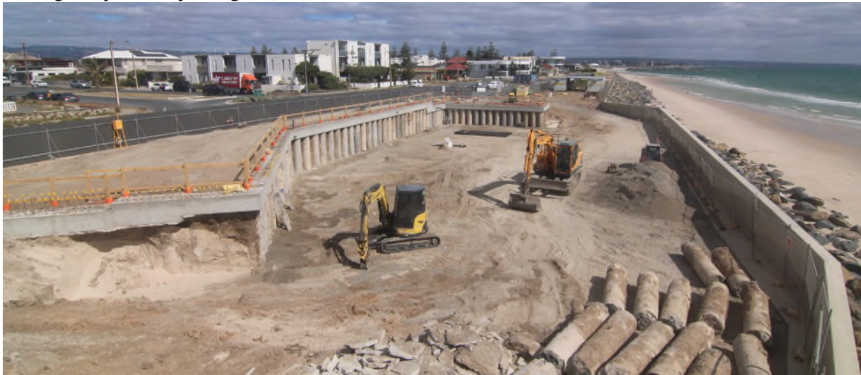
Bulking Out for Piled footings 15/12/2022
