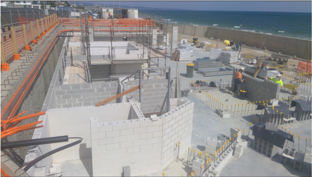
Lower Ground Blockwork – March 2023
