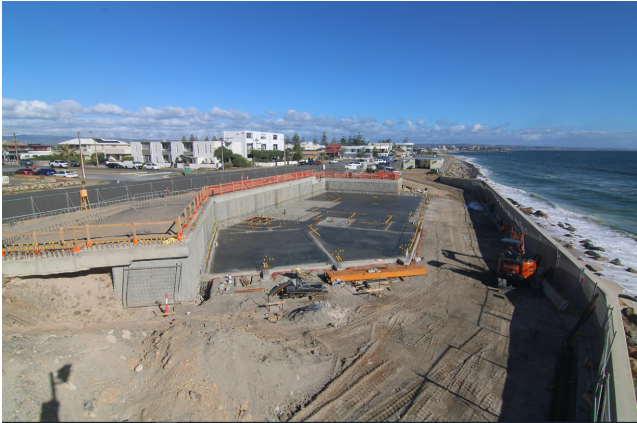
Lower Ground Concrete Slab – February 2023
