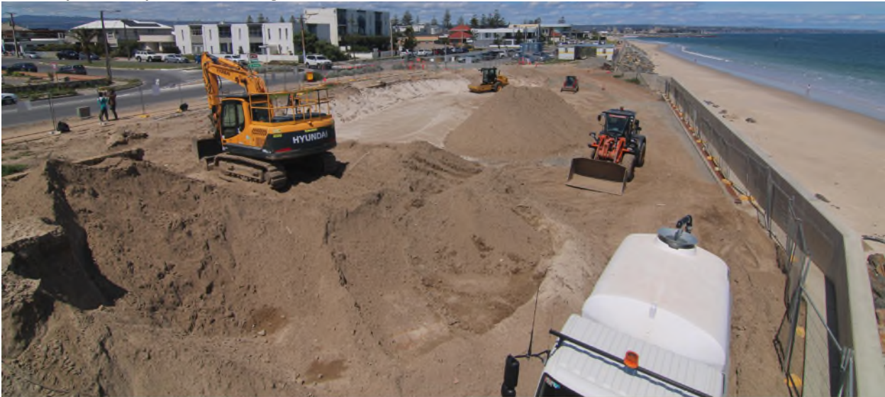
Site Preparation prior to Footing works October 10 2022
