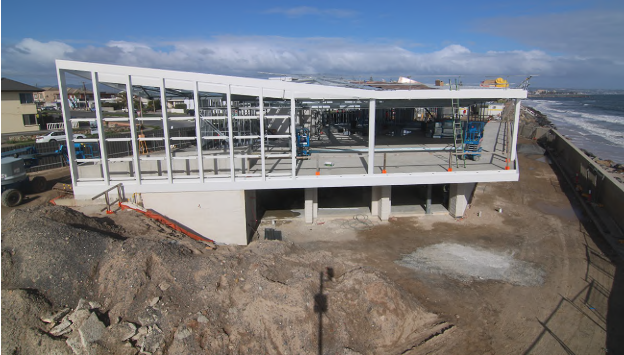
Structural Steel Completion August 2023
