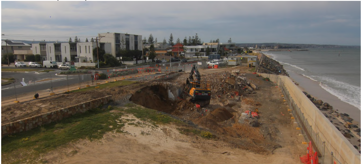
Demolition Complete September 20, 2022
