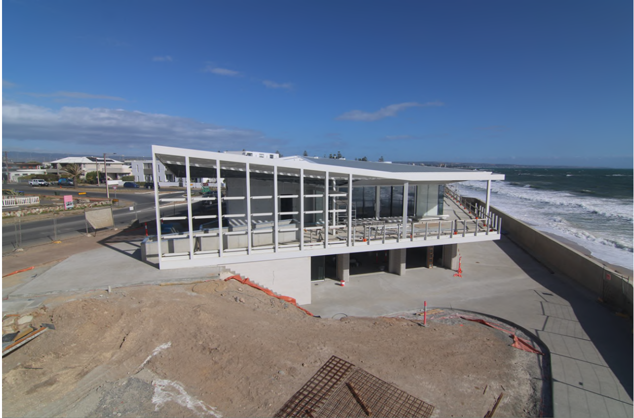
External Concrete works November 2023
