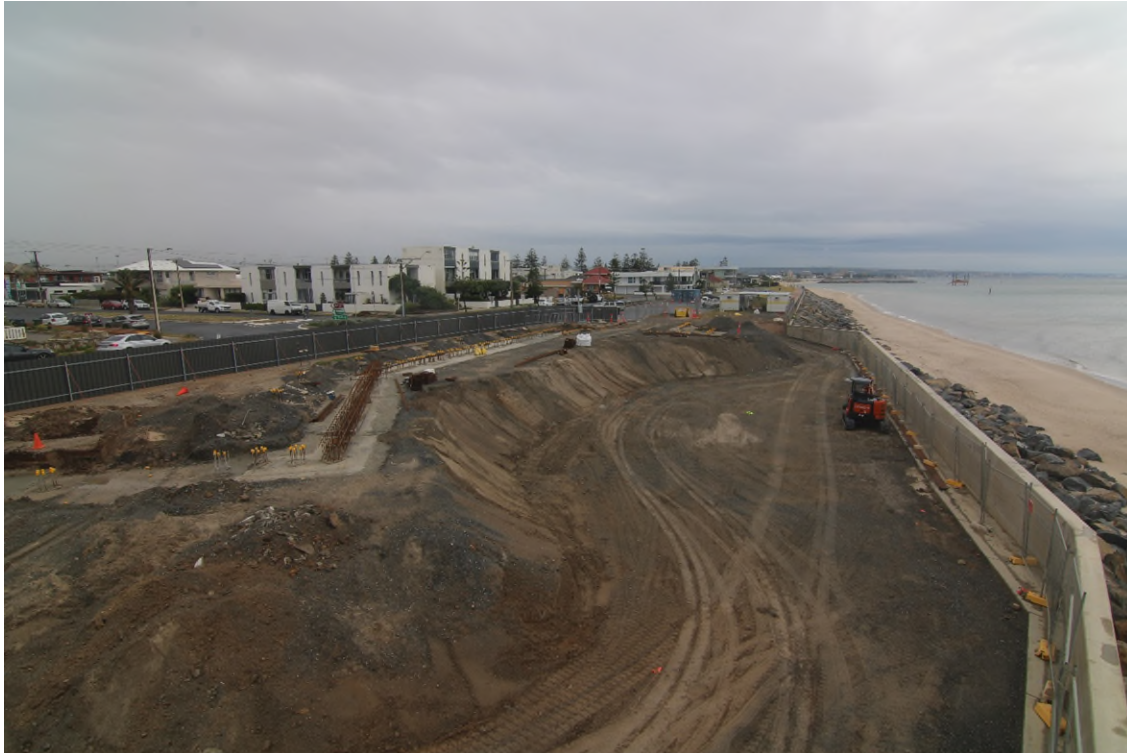
Piling complete ready for capping beam November 2022
