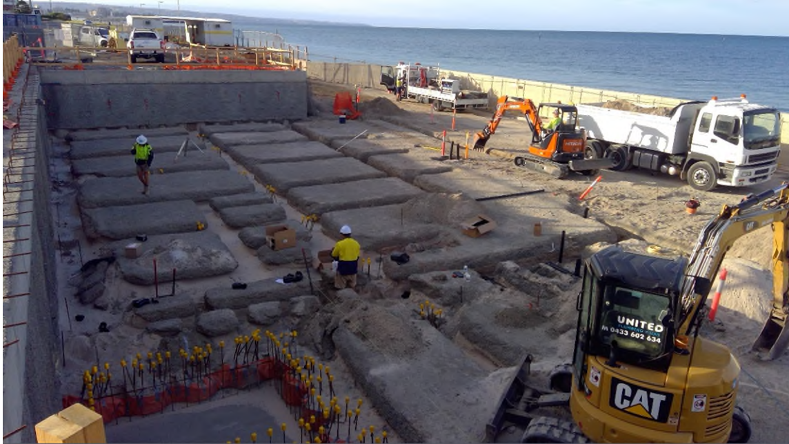
Lower Ground Footing works – January 2023
