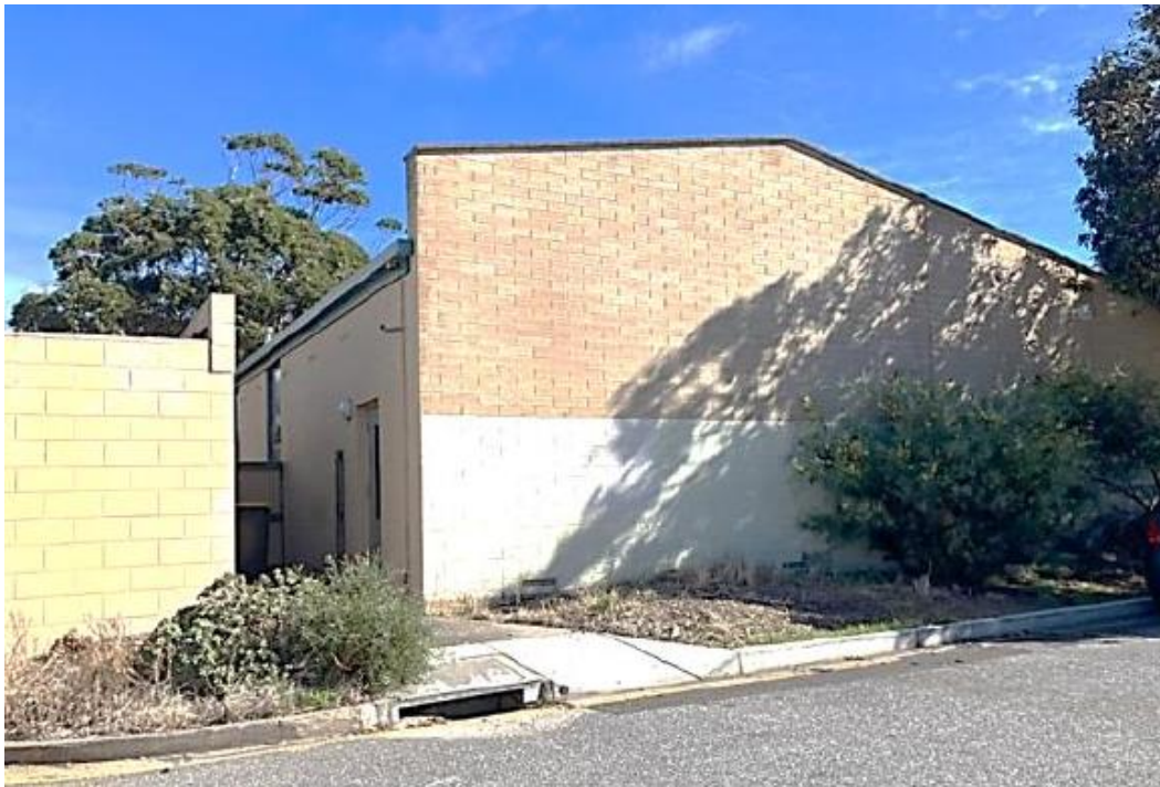
View from Sussex Street
