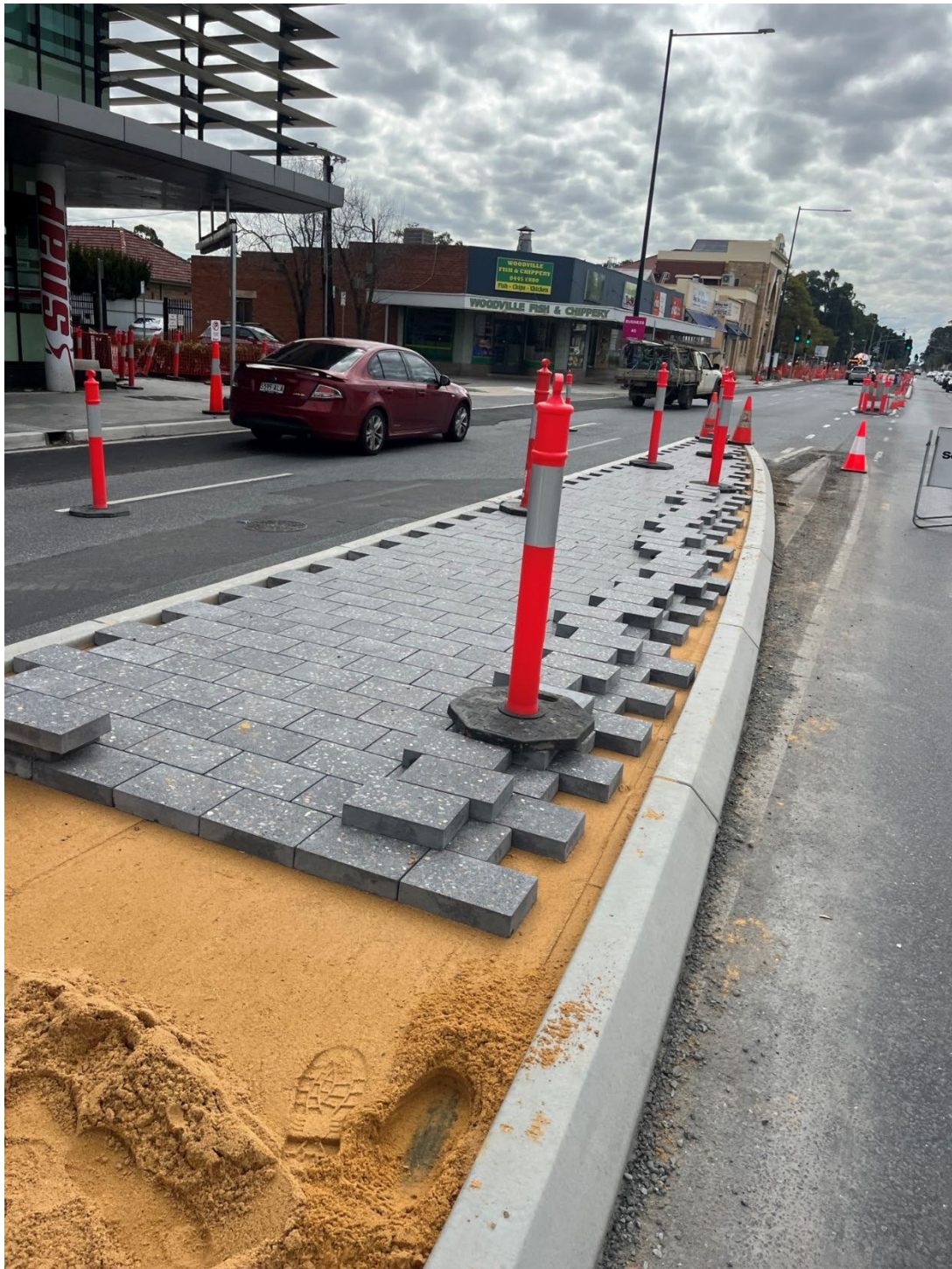
Paving commenced in Central median 21 August 2023
