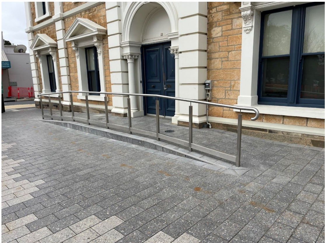
Town Hall Access Ramp - hand railing completed in July 2023
