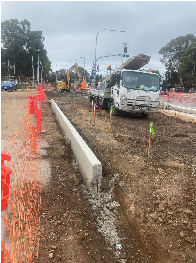
Civil works in progress between NNQ and Railway line 28 July 2023
