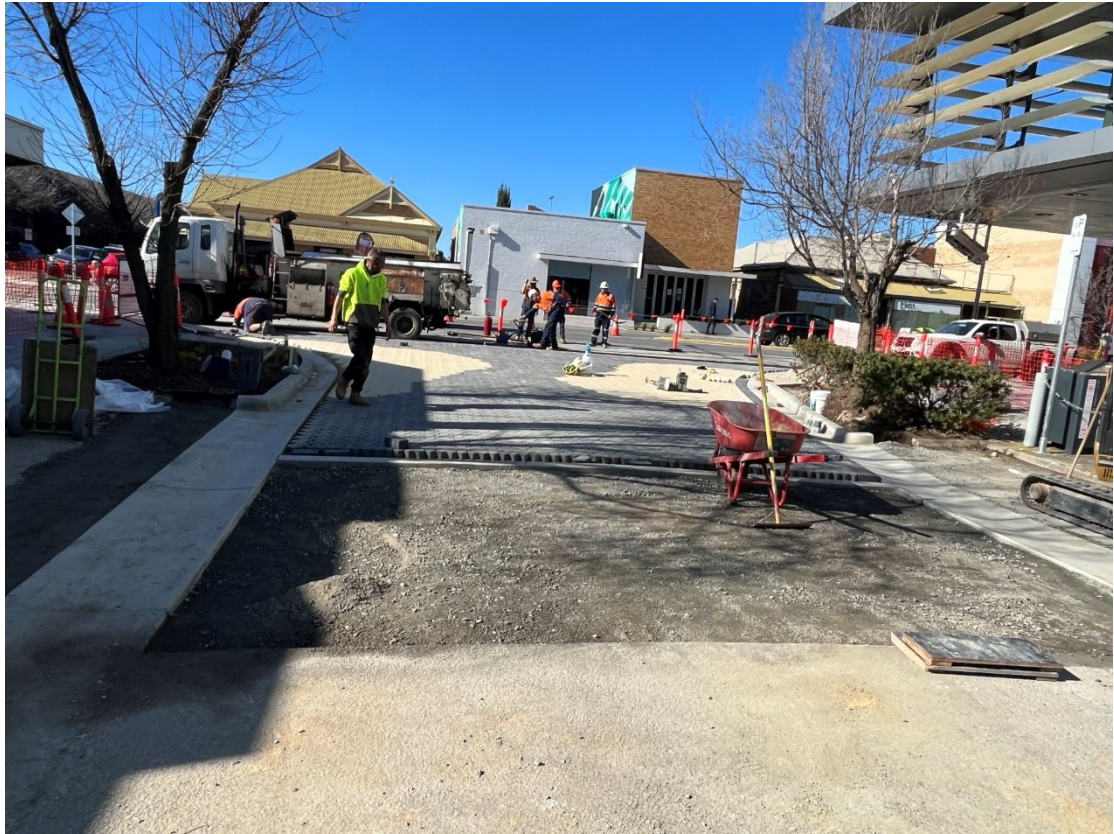
Aberfeldy Avenue intersection works 2 August 2023
