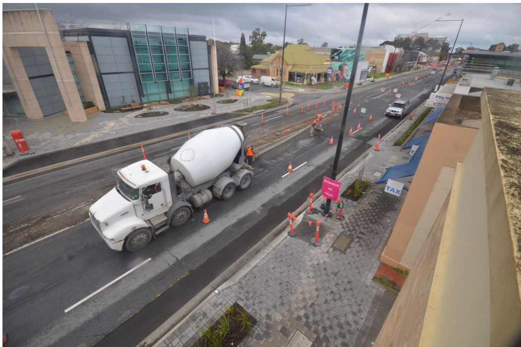
Median concrete works in progress - Taken by Time Lapse Camera 17 August 2023
