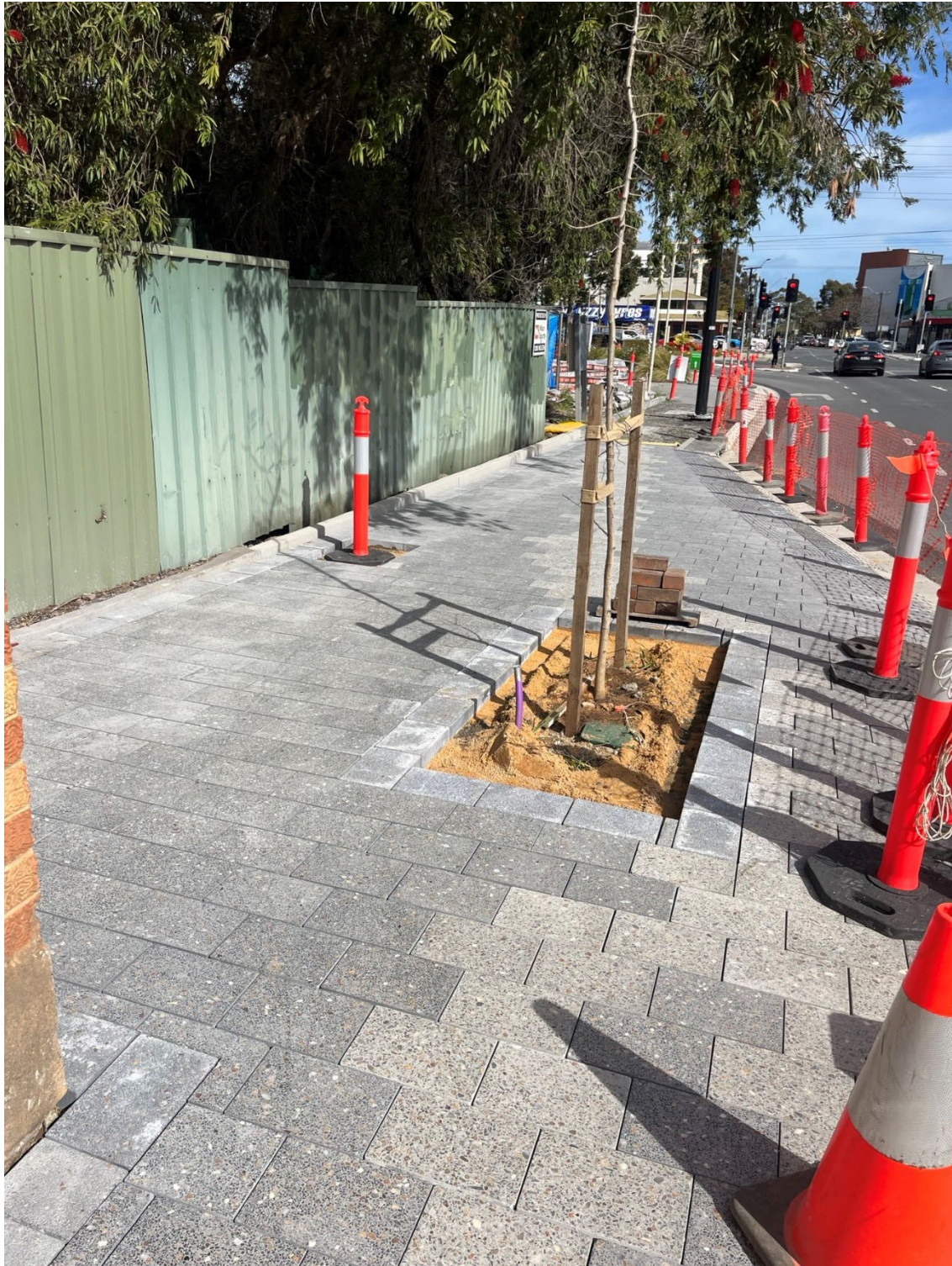
Paving and landscaping in front of car wash 17 August 2023
