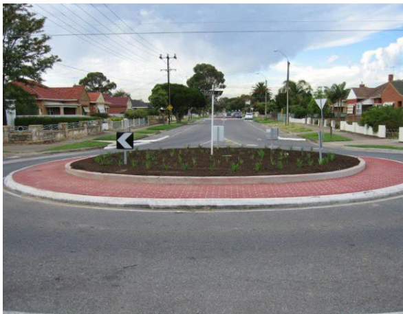
Greville Avenue, Flinders Park
