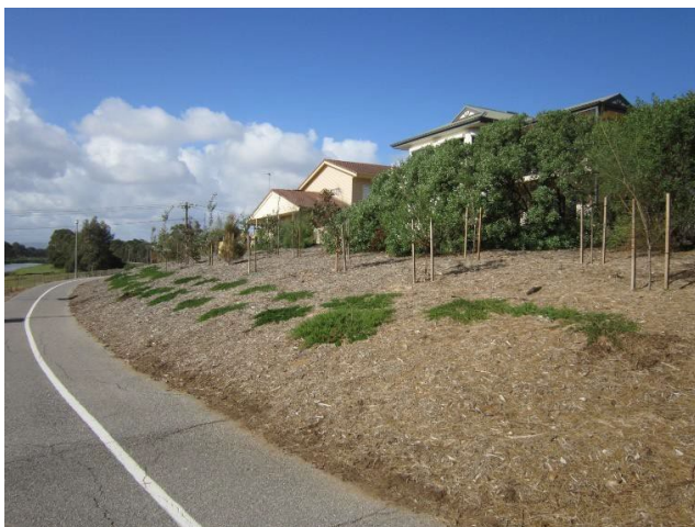
Example of a new habitat corridor along the River Torrens Linear Park at West Beach
