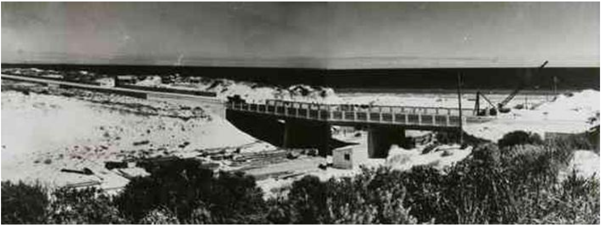
Figure 62 Construction of the bridge over the Torrens River outlet (B18651_9, SLSA)
