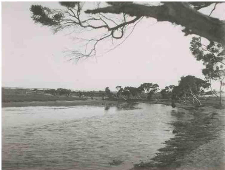
Figure 100 Patowalunga Creek, 1902 (B11752, SLSA)
