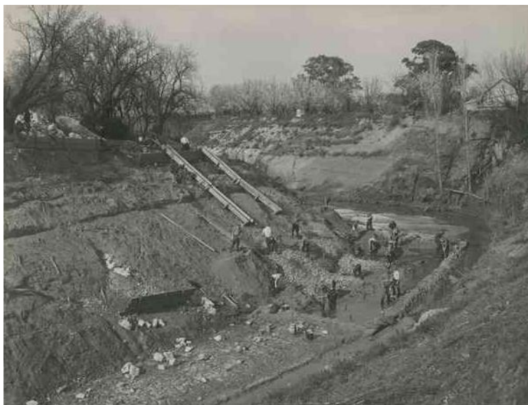
Figure 56 Improvements to Torrens River at Underdale, showing stone protection. 1938 (B11680, SLSA)
