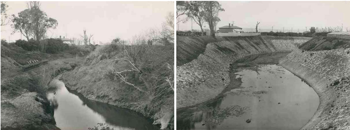
Figure 55 Torrens River, Lockleys, before 'improvement', 1937 (B11683, SLSA); Torrens River, Lockleys, after enlargement, 1939 (B11682, SLSA)
