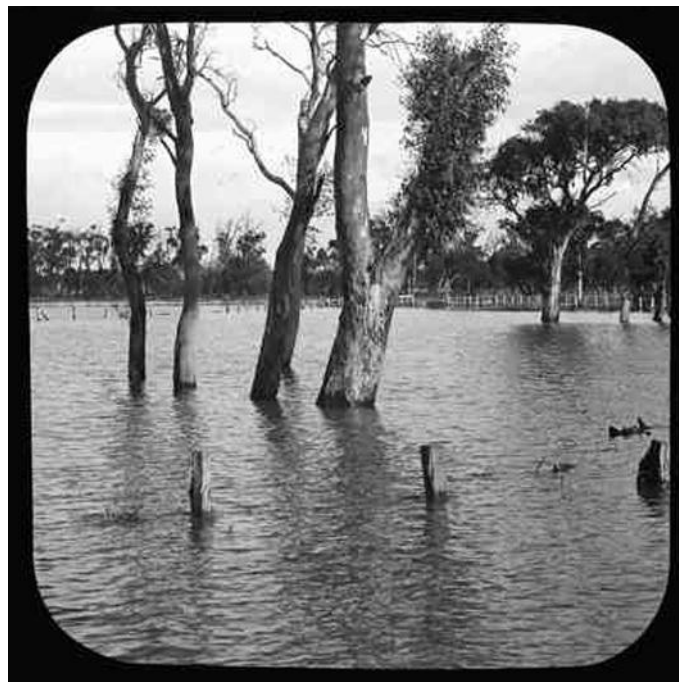
Figure 35 Floods on Henley Beach Road. Henley Beach, c.1910 (B64084, SLSA)
