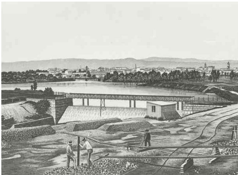
Figure 53 Torrens Lake Weir, c1880 (SLSA)
