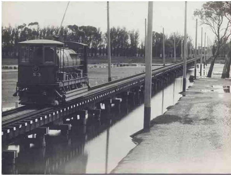
Figure 37 A 'scrubber' car on the viaduct (now Henley Beach Road), Reedbeds, Fulham (B70935_16 (SLSA)
