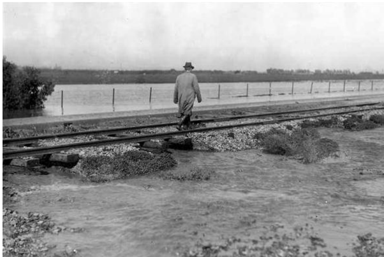
Figure 42 Floods by the railway track at Grange, 1923 (PRG 280/1/41/170, SLSA)
