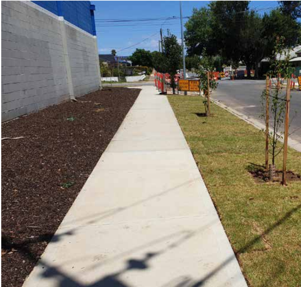
| New May Street footpath and verge widening
