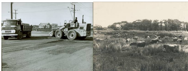
From left: Road construction Fulham Gardens Tapleys Hill Road and Marlborough Street 1960s, cattle grazing in the reedbeds c.1910
